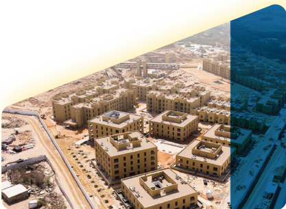
AMAALA STAFF VILLAGE PROJECT
