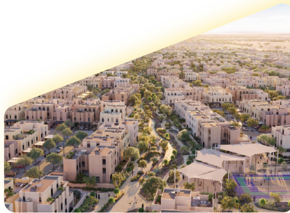
ROSHN VILLAS PROJECT
